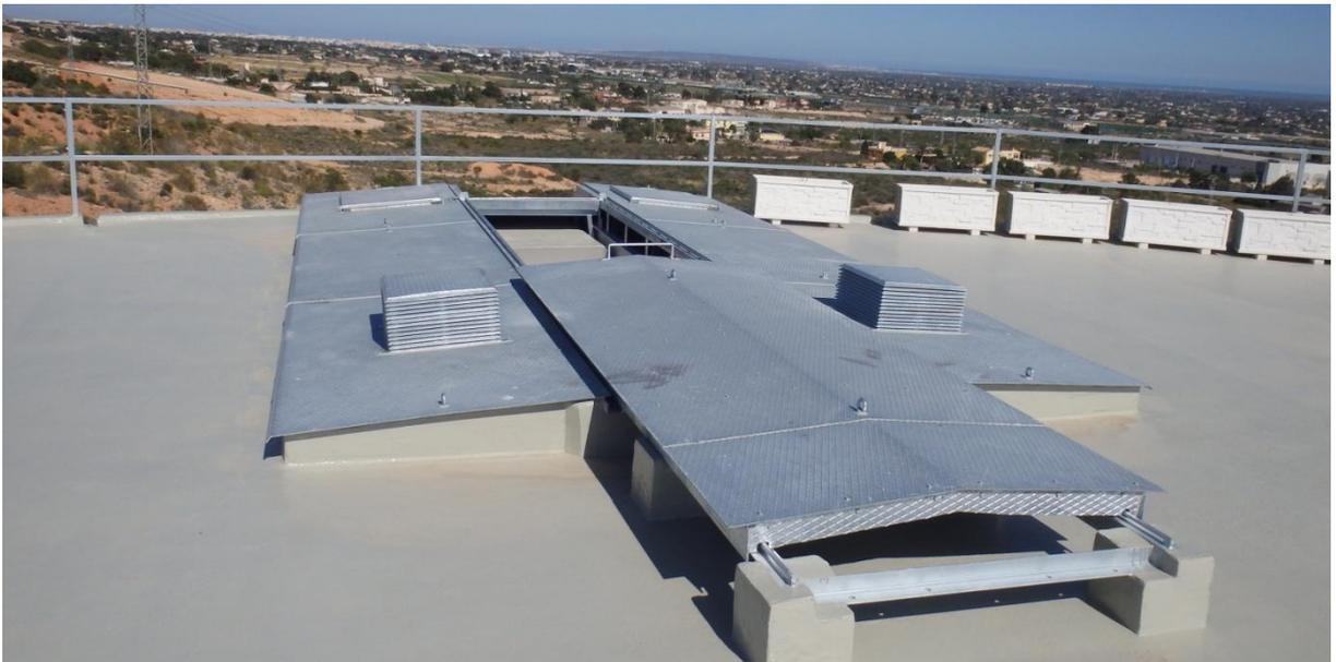
ACCESO MEDIANTE TRAMPILLA CORREDERA PARA ACCESO AL INTERIOR DE LA CÁMARA
